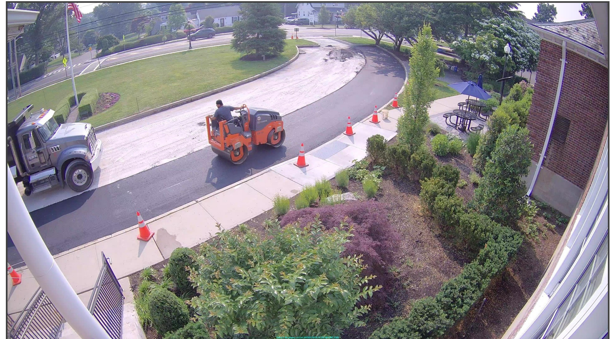
Re-paving the Broadway Circle
