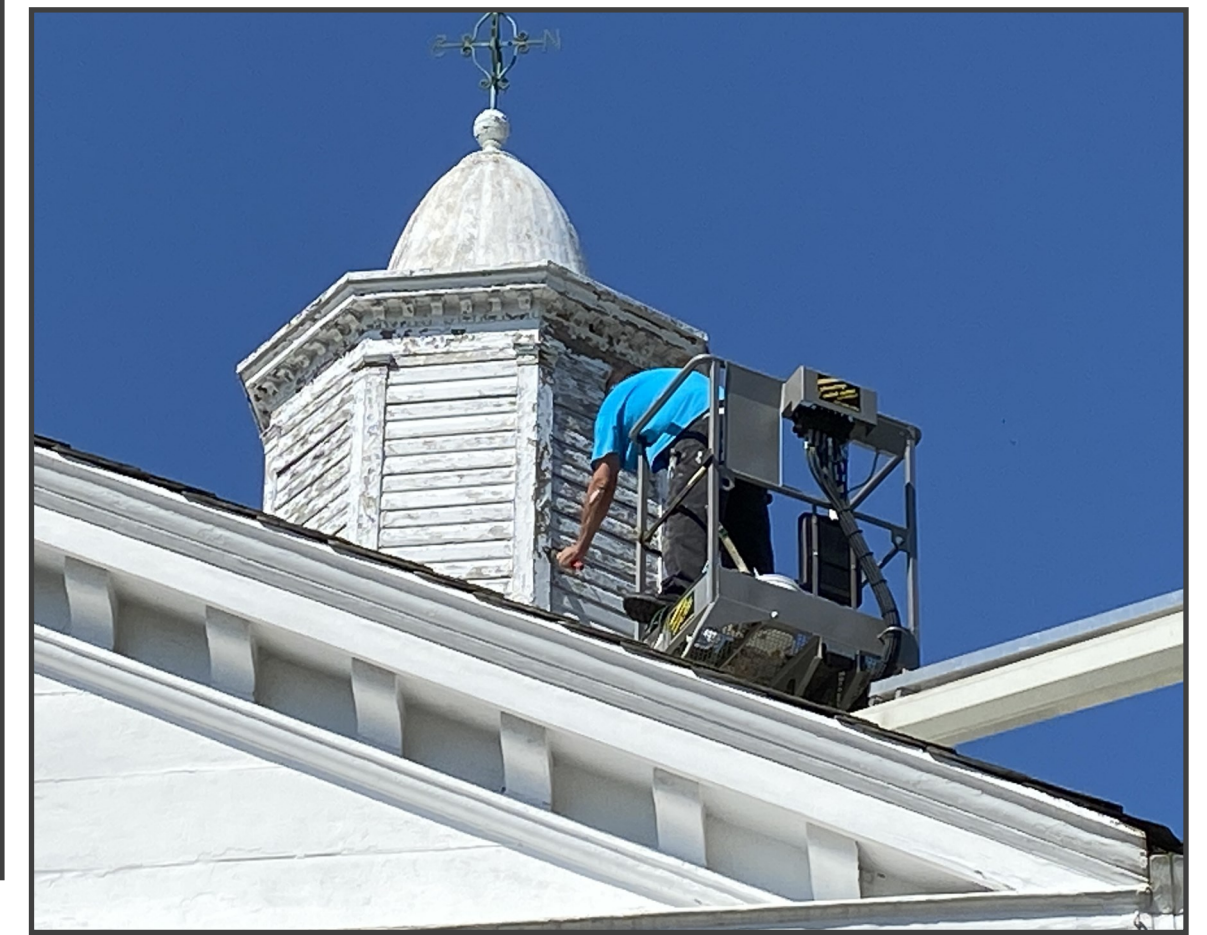
Repairs Are Made to the Broadway Cupola
