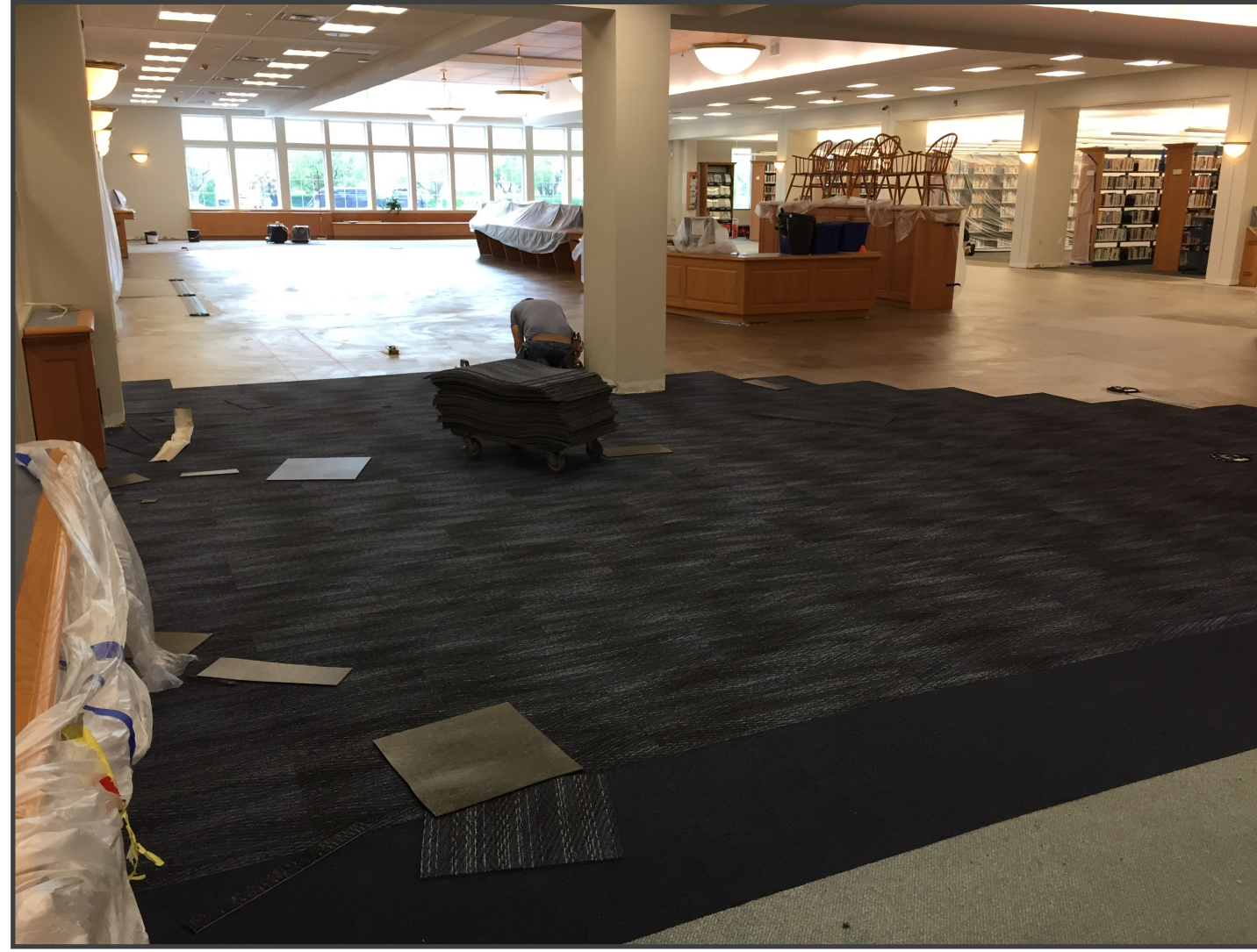
Carpeting in the Reference Room
