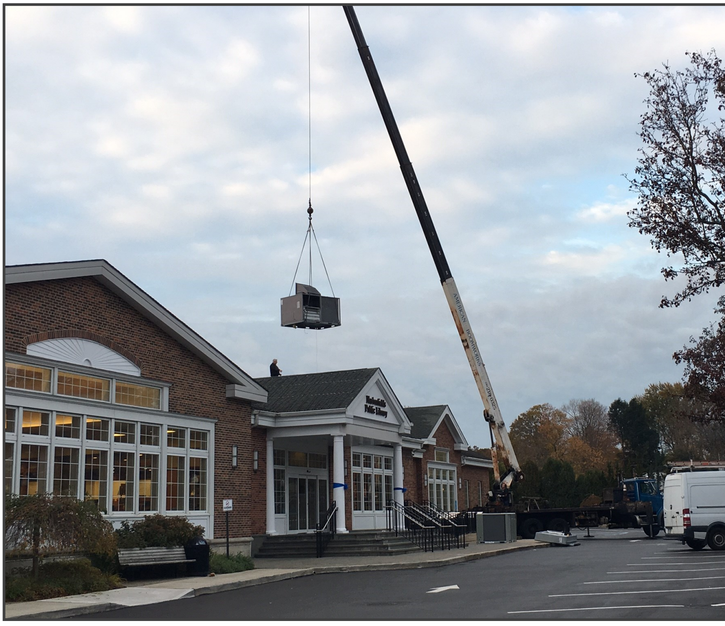
New Roof-Top HVAC Units
