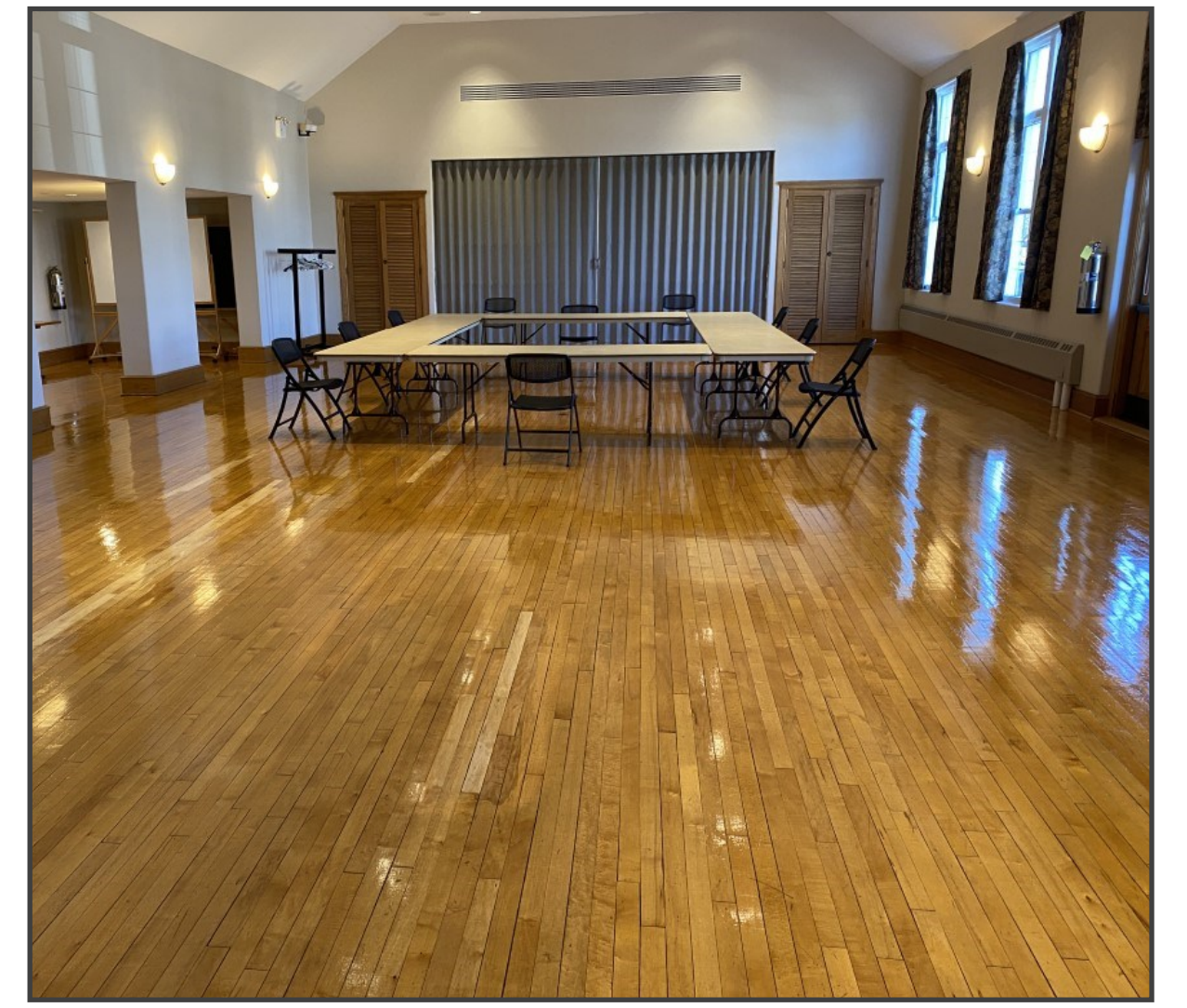
Repair and Refinish the Original Flooring in the Community Meeting Room
